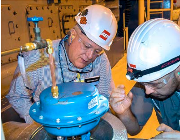
Assistant Maintenance Director John Wygant (left) passes along some of his 35 years of valve maintenance knowledge to a young coworker.
